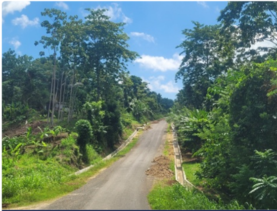
Type 5 Open drain on both sides of the road on New Britain Highway, East New Britain
