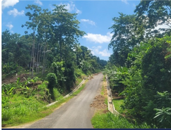
Type 5 Open drain on both sides of the road on New Britain Highway, East New Britain
