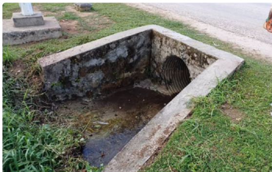
Culvert Cleaning and drainage works on Momote Road, Manus
