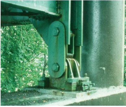
Pin and link bearing
