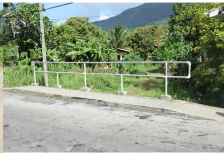
Steel handrail and concrete kerb
