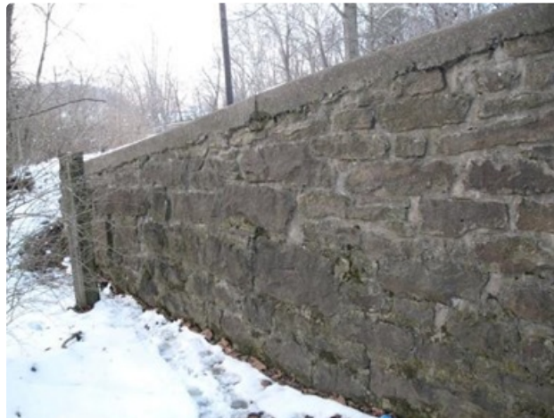
Freestanding and splayed wing wall
