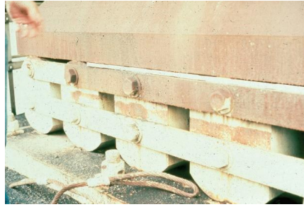
Segmental rocker nest bearing
