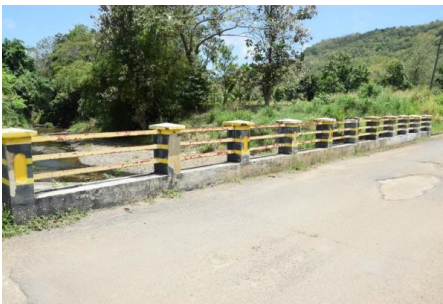
Concrete and steel barriers
