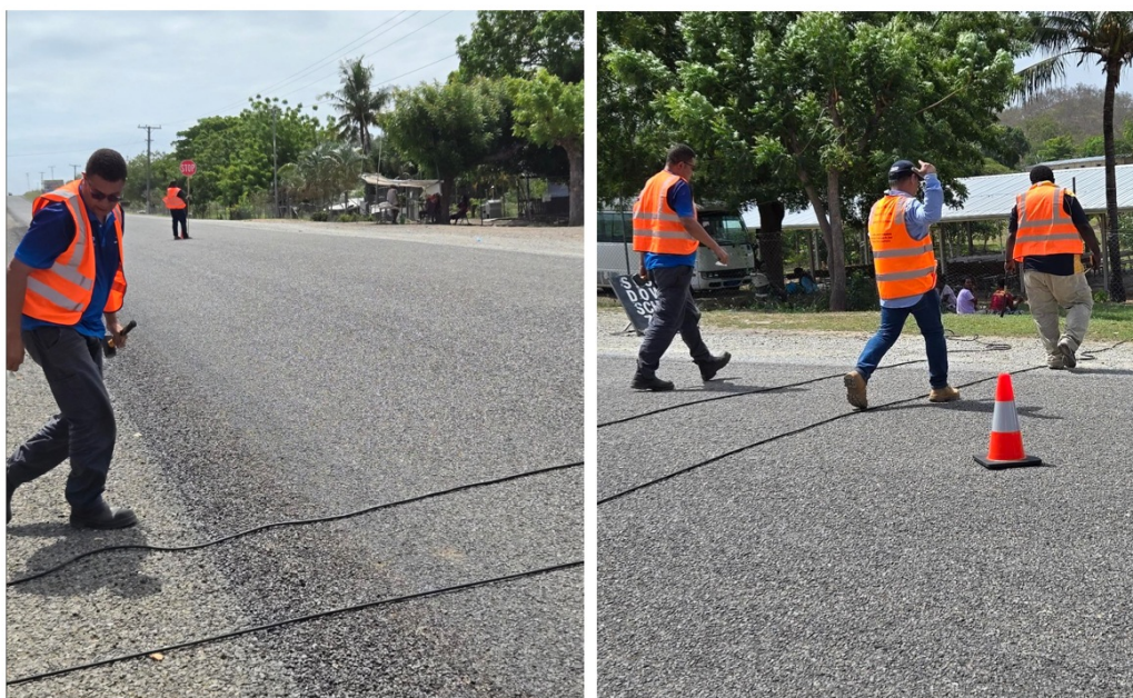
Typical example of setting out details of MetroCount device during installation and uninstallation. Note Dayglow vests, STOP/SLOW signs and road cones to help manage safety on site
