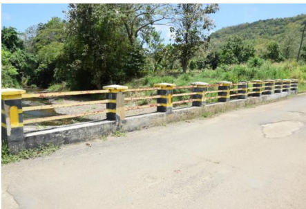
Concrete and steel barriers
