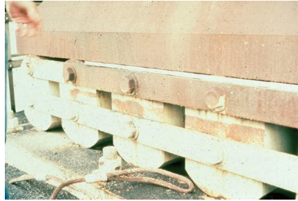
Segmental rocker nest bearing
